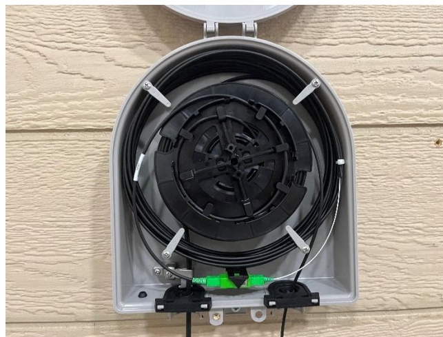
Figure 3 CraftSmart Deploy Reel TAP with FLEXdrop Deploy Reel
