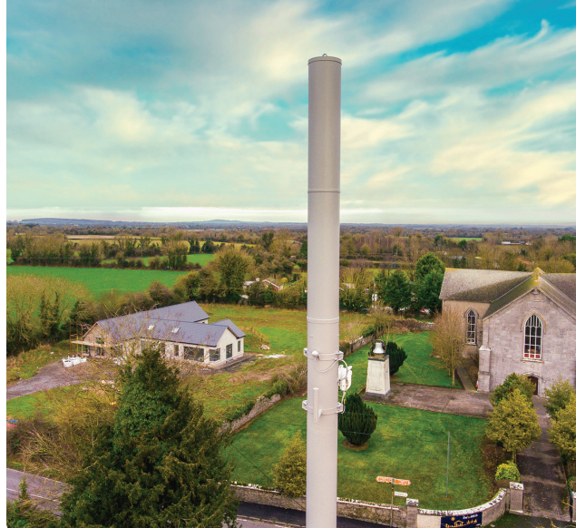
FIGURE 2. Pictured is a multi-band, tri-sector antenna deployed by Cellnex in the village of Vicarstown, County Laois, Ireland. Photo source: Alpha Wireless
