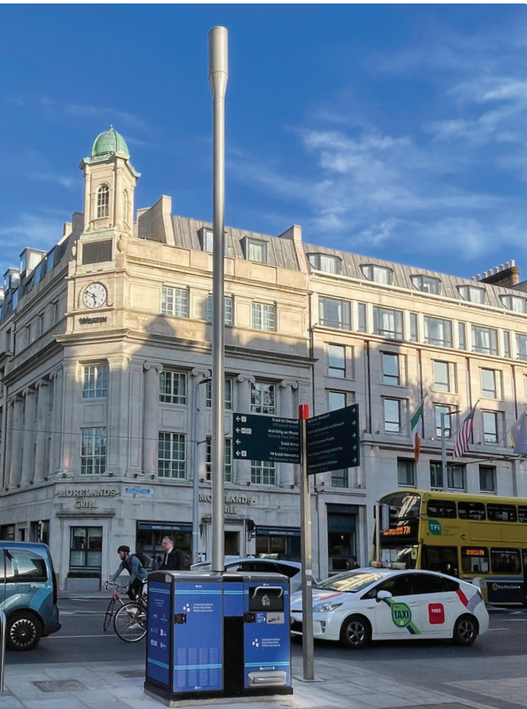
FIGURE 1. New small cell deployments in Dublin included a smart connected waste and recycling bin, the Big Belly Telebelly, which conceals radios, power, and transmission equipment discreetly within a sensor-equipped enclosure.
