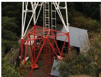
FIGURE 1. Telecom tower with a solar power plant at a remote island in Nicaragua. (Source: THEnergy)
