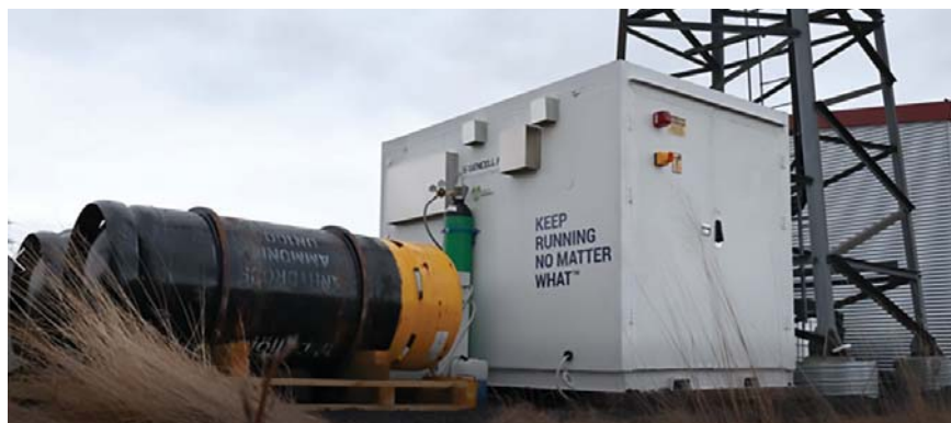
FIGURE 2. Fuel cell at a telecom tower in Iceland. (Source: GenCell)
